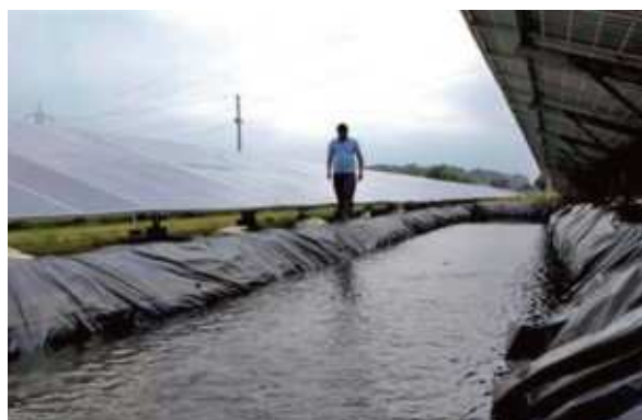
Aquavoltaics site in Bhaloj, Rajasthan.
