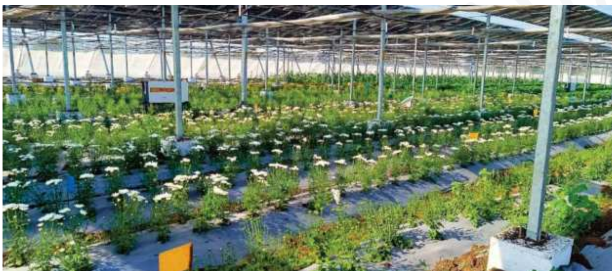
Agri-PV installation. © SunSeed APV.
