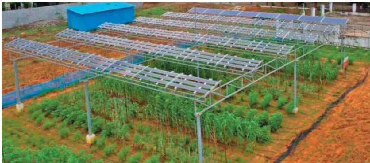
Semi-transparent PV panels installed at Seed Research and Technology Centre (SRTC), PJTSAU, Rajendranagar, Hyderabad. © Renkuba.
